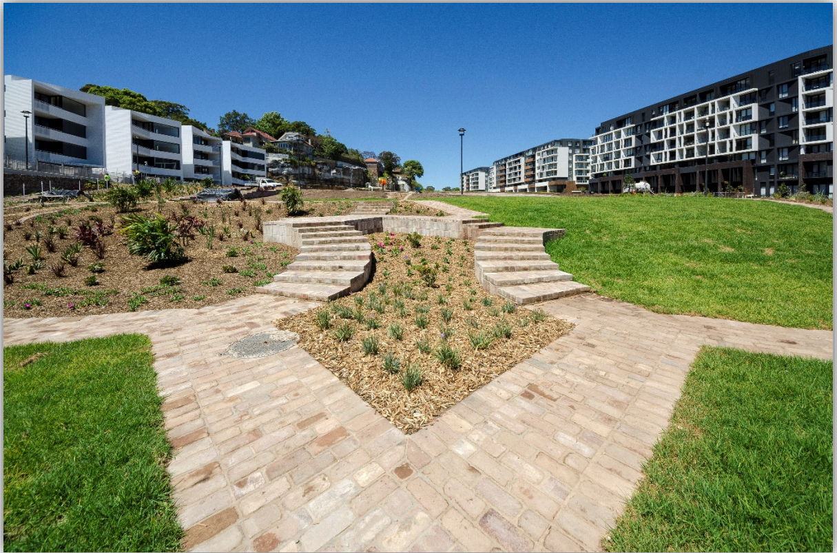
Images of park under construction (October 2016)
